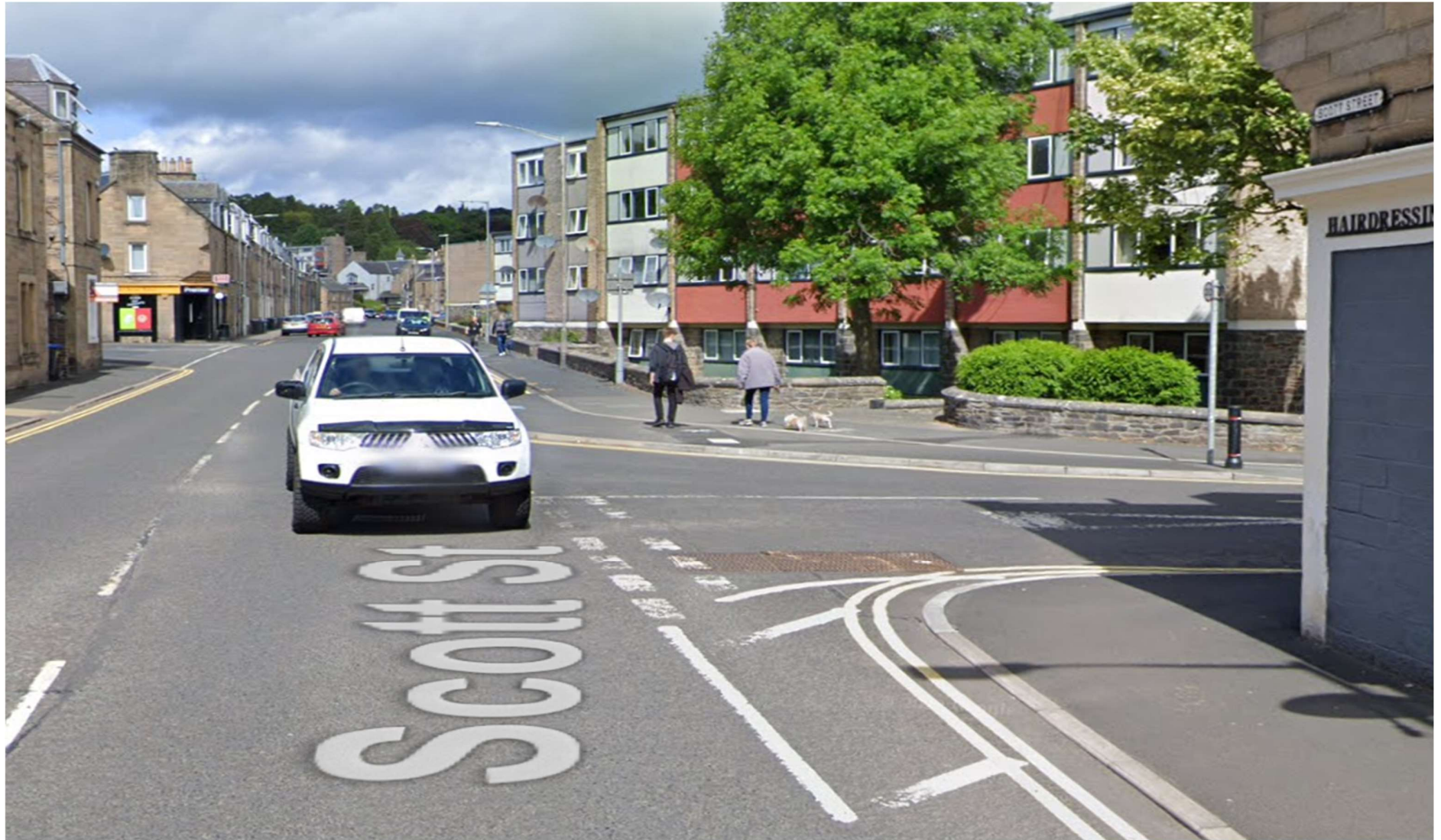
Figure 6: Road markings at junction to assist with visibility - Galashiels
